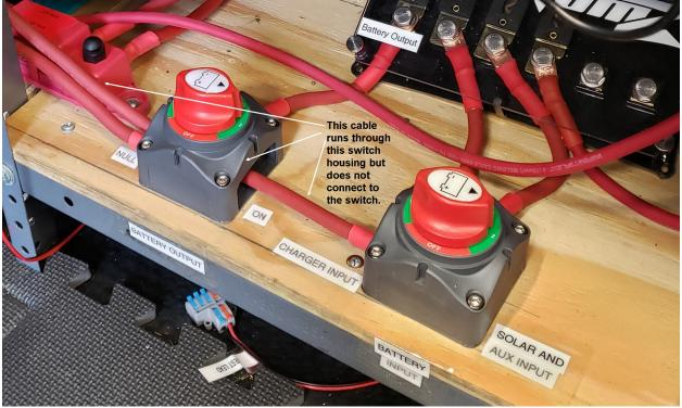
The cable runs to the 12V system positive bus bar which connects to the positive terminal of the JITA 12V 200Ah Plus LiFePO4 Battery with Built-in 200A BMS.
