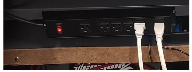
To charge the LiFePO4 battery using shore power, plug in a LiFePO4 charging unit into this power strip, then connect the leads to the AUX Positive and Negative busbars.
