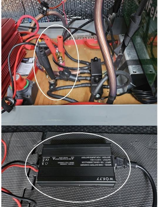
The AUX positive busbar connects through a 60A ANL fuse to position #2 of **Switch #2**. To use shore power charging, **Switch #2** and **Switch #4** should both be set to position #2.
